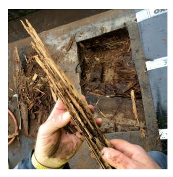
The boards and edge timbers in this area were wet and one area was found to be heavily infested with larvae.
