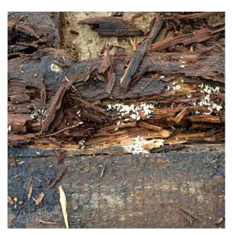
In areas there was no support at all for the asphalt – which was hanging in mid span. The roof was patched back as far as was possible. However, there is a real danger that as the roof dries out under the patch,
