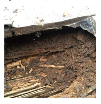
"The work revealed that the area along the edge of the roof is profoundly rotted away – reducing to a soil-like consistency.
